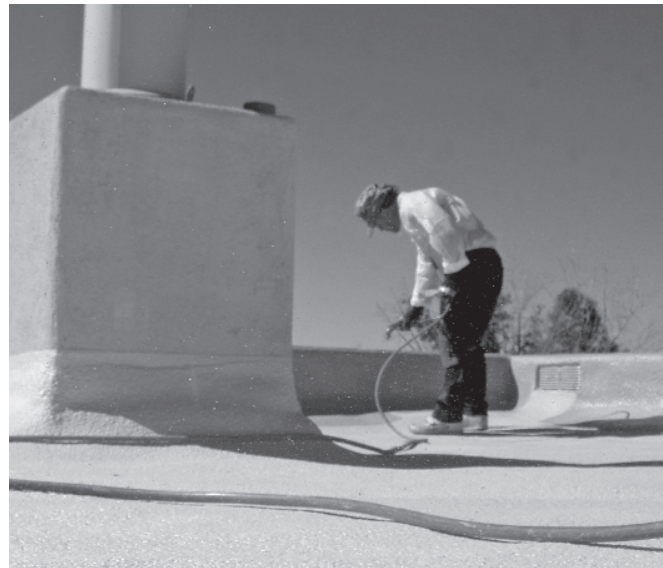
Figure 4. Another option to protect SPF roofing from ultraviolet light is a sprayed-on coating. Most roof coatings last for 10 to 15 years before they need to be renewed. [Photo credit: Thermal Coatings and Insulation]
