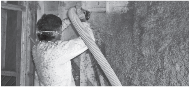
Figure 6. A comparison of the airtightness of 182 cellulose-insulated houses and 684 fiberglass-insulated houses revealed that the cellulose-insulated houses are significantly more airtight.
