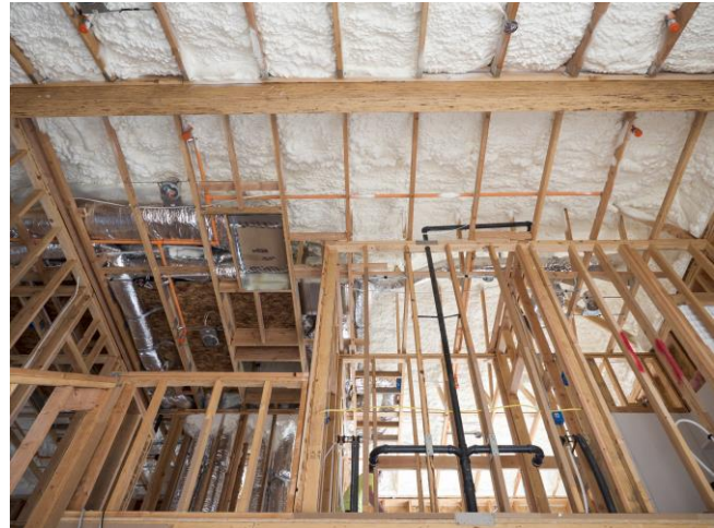
Open-cell spray foam installed below roof deck
