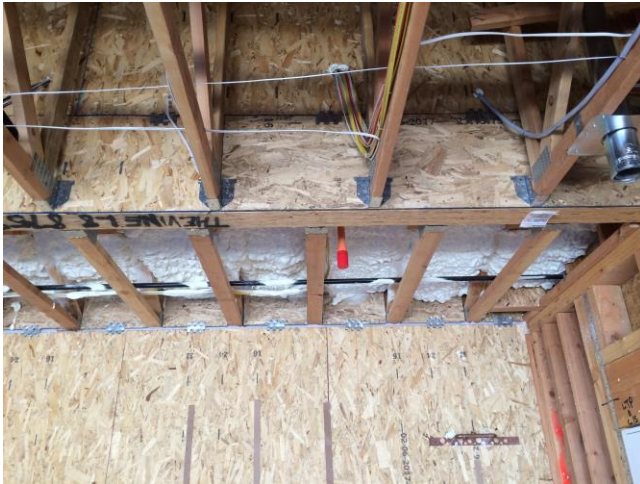
Open-cell spray foam installed at rim joist Figure 9. Photos of homes sealed under Option 1
