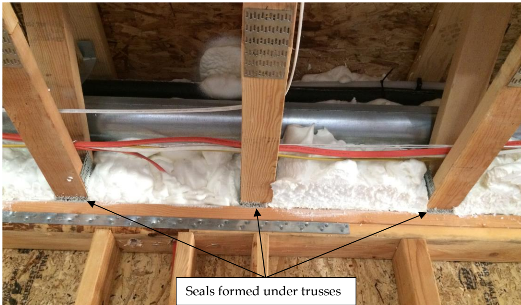
Figure 5. Photo of seals formed below each truss on first floor
