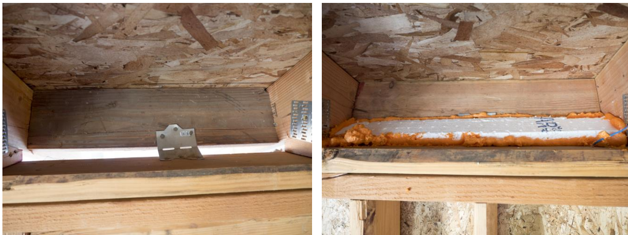
Figure 8. Gap at eave prior to sealing (left) and after sealing with ridged foam and can foam (right)
