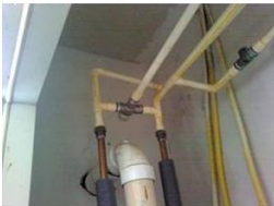
Water and space heating uninsulated pipes in a resident unit
