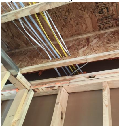
Foam seal electrical penetrations to garage
