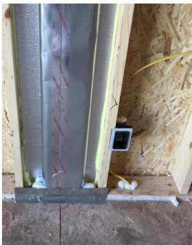
Duct and electric penetration thru exterior wall base plate
