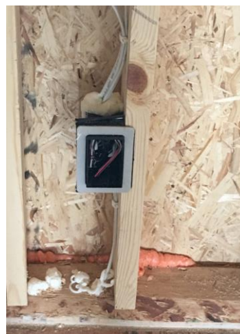
Air-tight electric box at exterior wall; caulk base plate/floor joint
