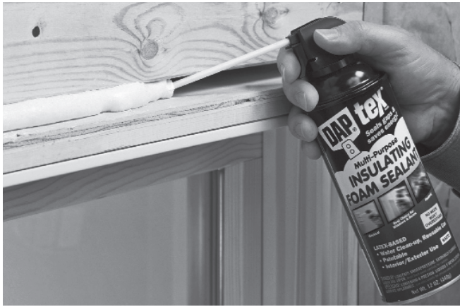
Figure 7. Unlike one-component urethane spray foam, DapTex foam cleans up with soap and water.
